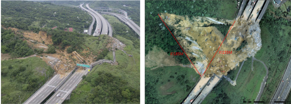
Figure 1 The National Highway No. 3 landslide Aerial Photo (TGS, 2011)
