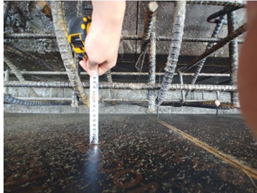
b) wall thickness / cover depth
