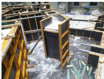
a) Corner joint specimen
